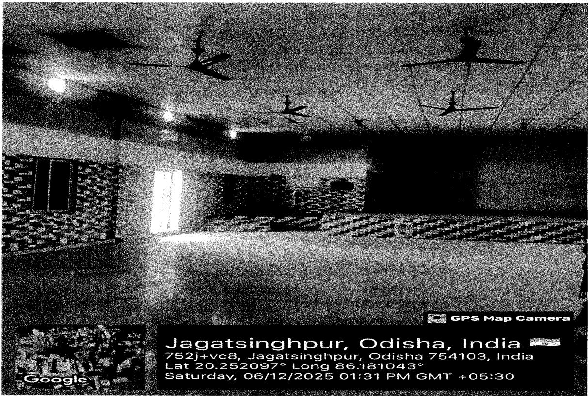
Proposed Site for Renovation of Town Hall at Panisalia in Ward No.16
