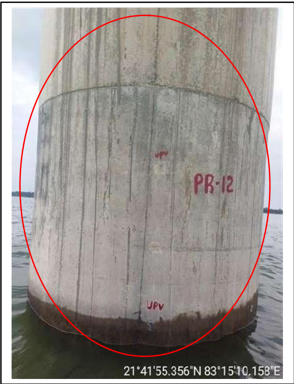
Picture-3 & 4: Cracks on pier surface
