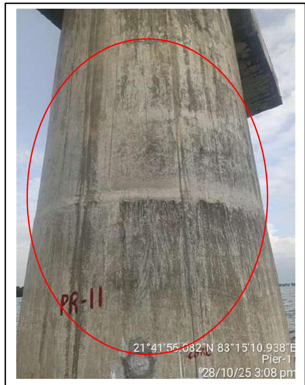
Picture-2: Cracks on pier surface
