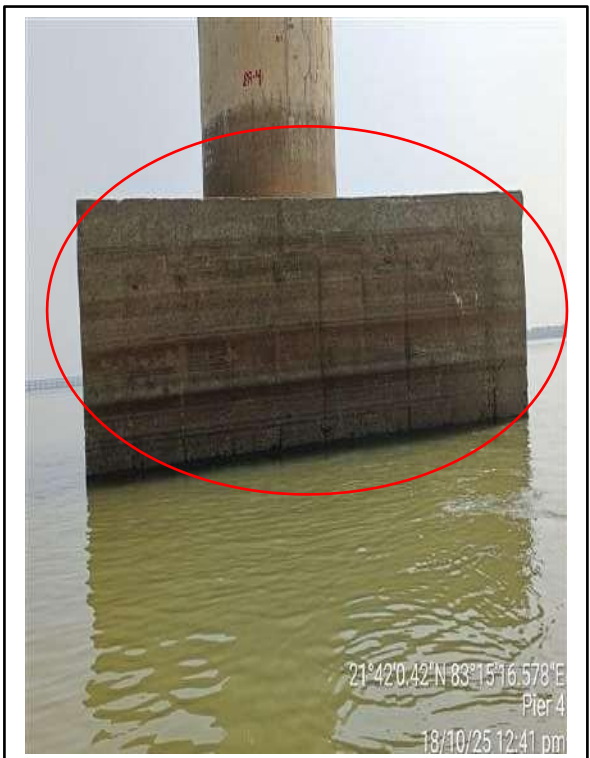
Picture-7 & 8: Cracks on pile cap surface
