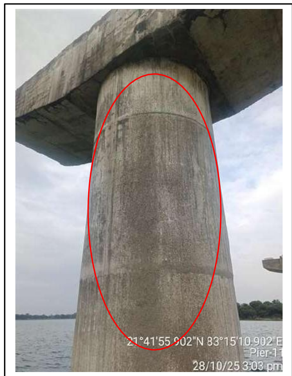
Picture-3 & 4: Cracks on pier surface
