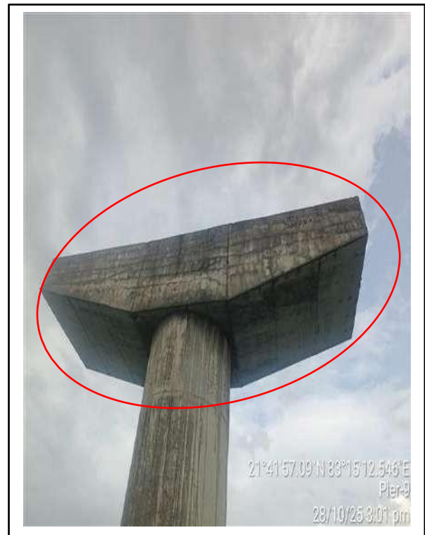
Picture- 5 & 6: Minor cracks, leaching & efflorescence on pier cap.
