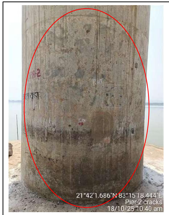
Picture-2: Cracks on pier surface.
