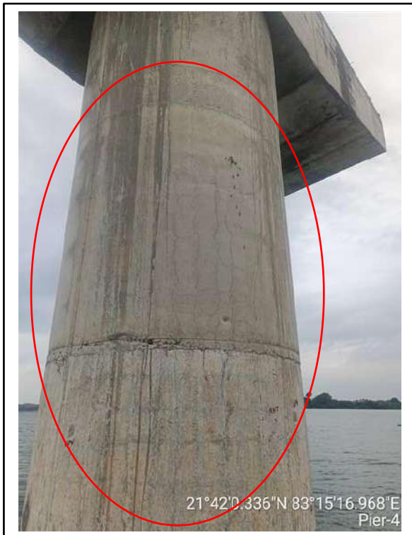
Picture-3 & 4: Cracks on pier surface
