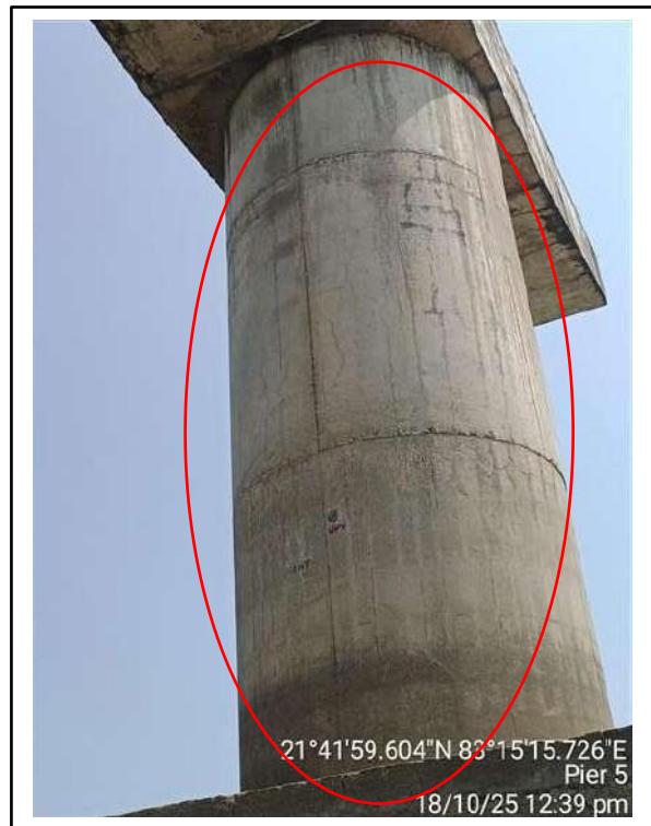
Picture-2: Cracks on pier surface
