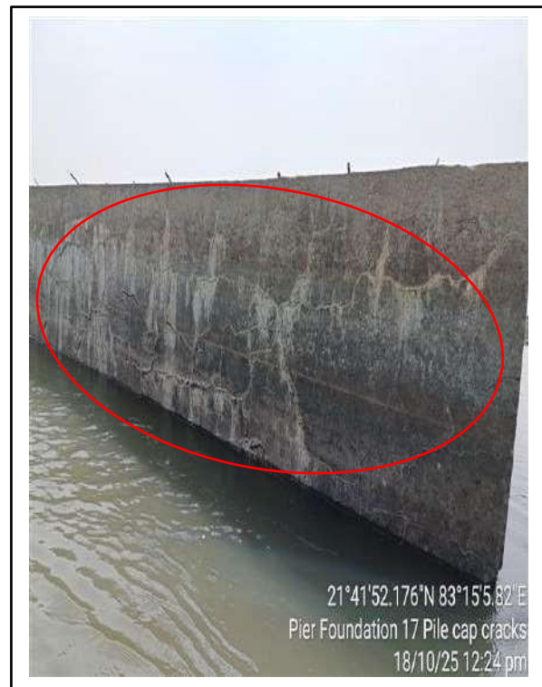
Picture-2: Cracks on Pile cap side face.
