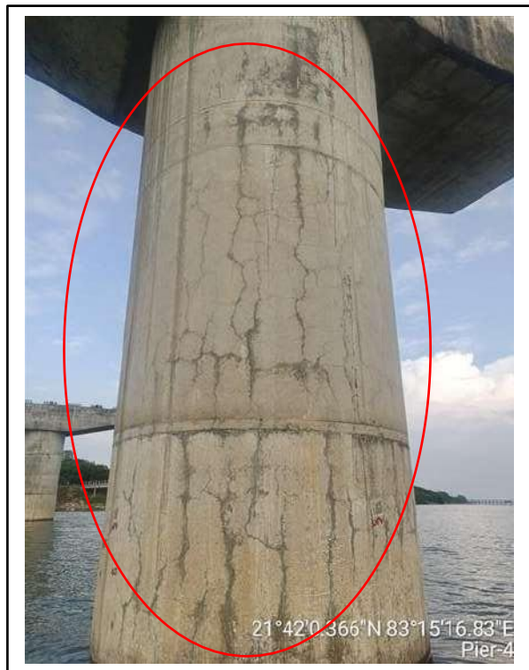
Picture-3 & 4: Cracks on pier surface
