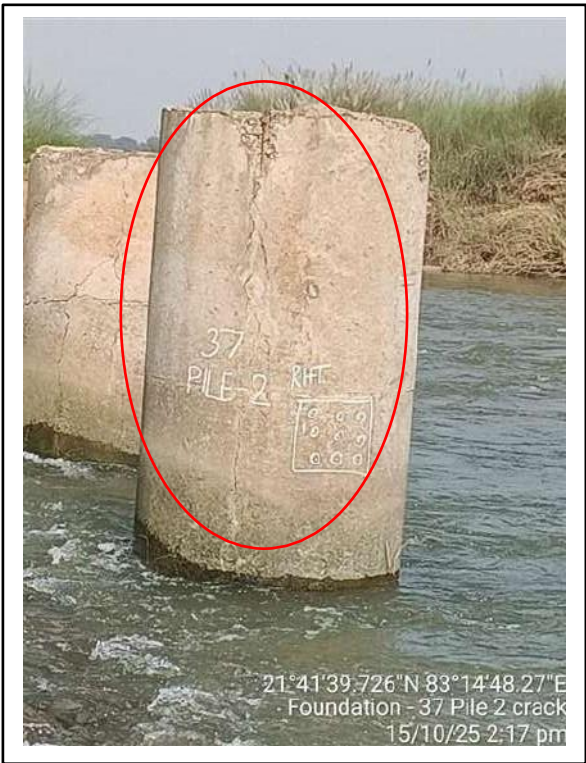
Picture-3 & 4: Cracks on pile concrete
