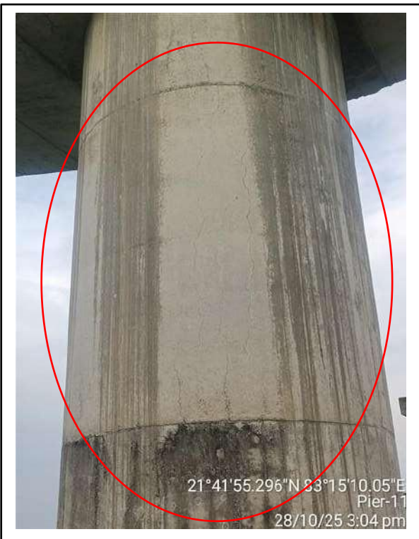
Picture-3 & 4: Cracks on pier surface
