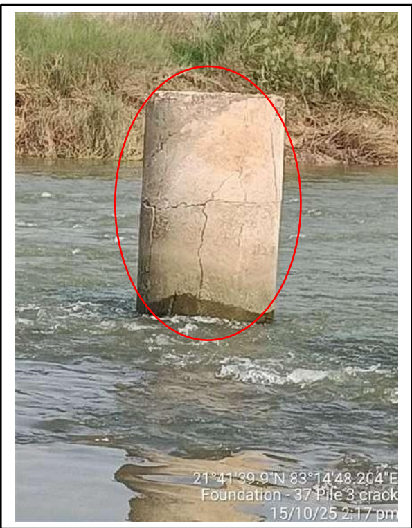
Picture-3 & 4: Cracks on pile concrete
