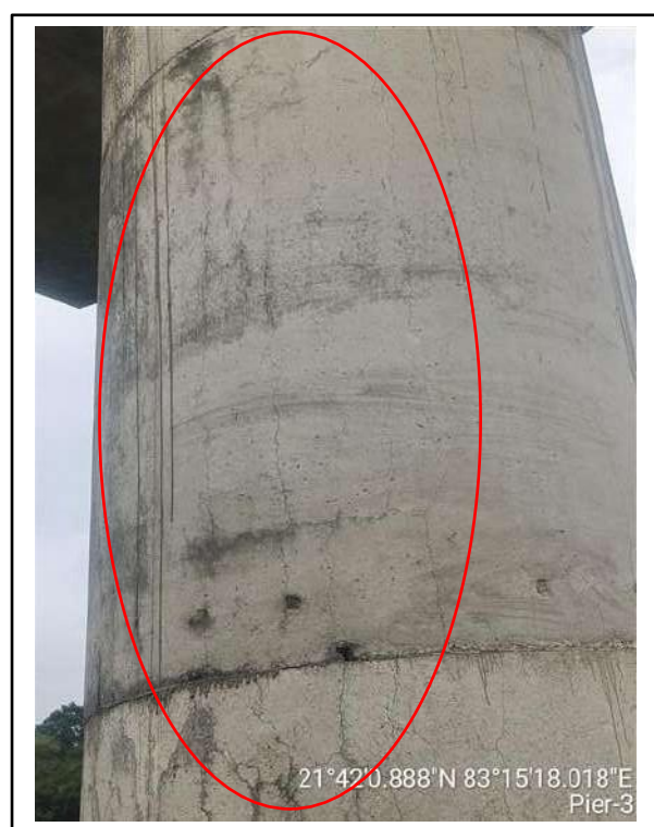
Picture-3 & 4: Cracks on pier surface
