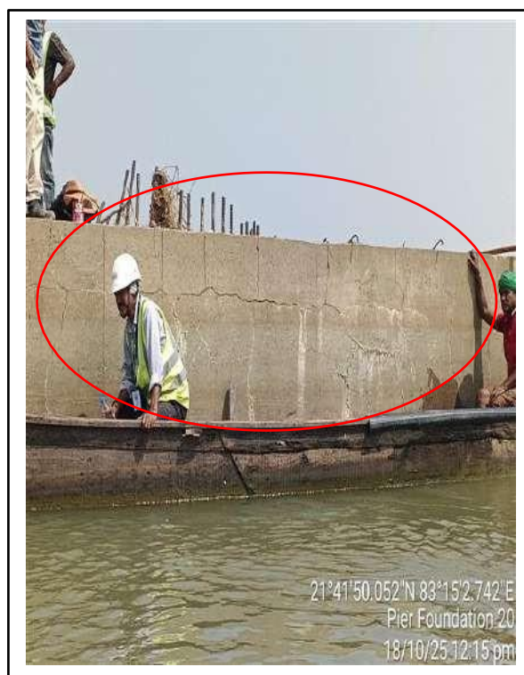
Picture-2: Cracks on pile side face.
