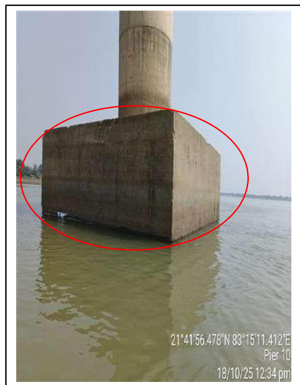
Picture-7 & 8: Cracks on pile cap surface
