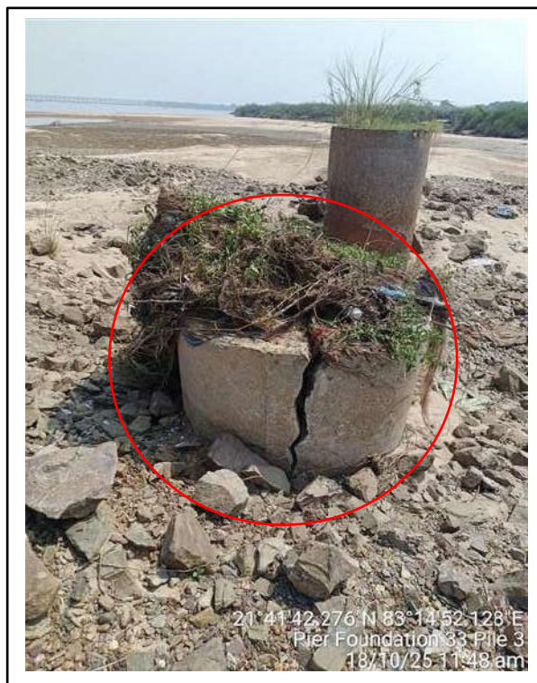
Picture-3 & 4: Cracks and debris on pile concrete
