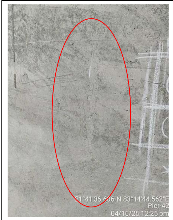
Picture-3: Cracks on pier surface.
