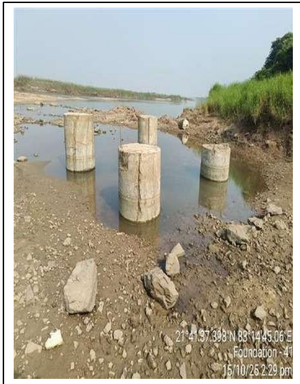
Picture-1: Piles foundation – 41 view
