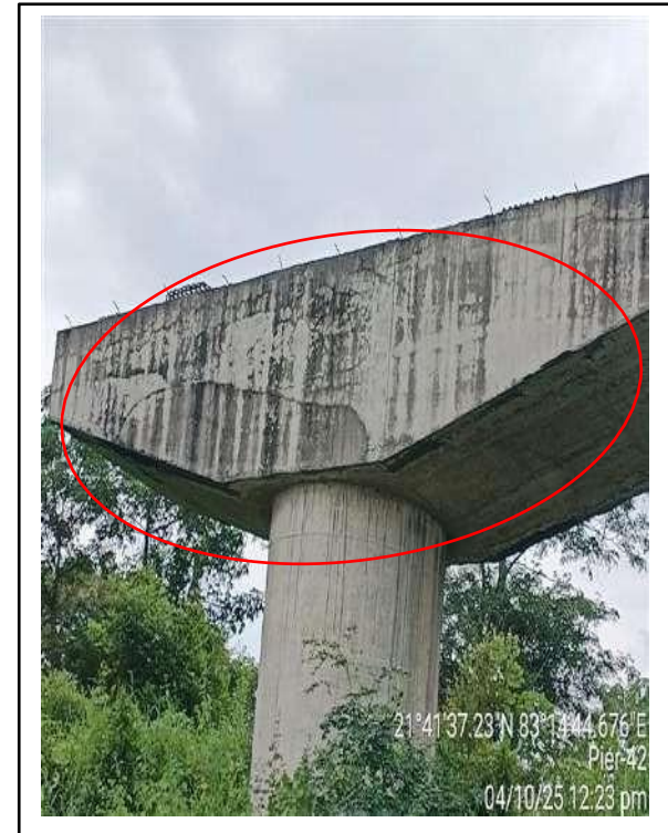
Picture-4: Minor cracks & leaching on pier cap
