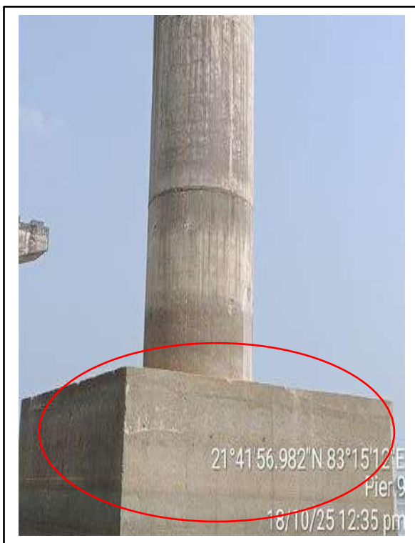
Picture-7 & 8: Cracks on pile cap surface
