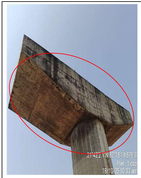
Picture-4: Leaching & Minor cracks on pier cap.
