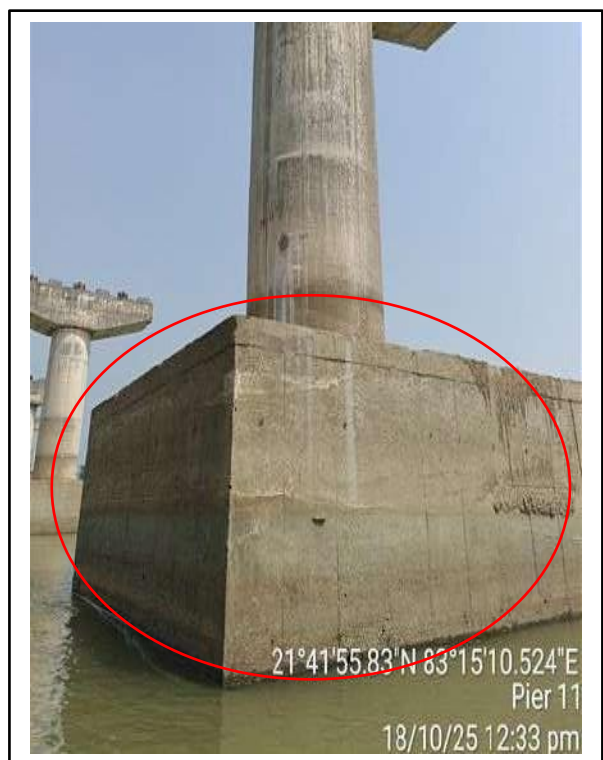
Picture-7 & 8: Cracks on pile cap surface
