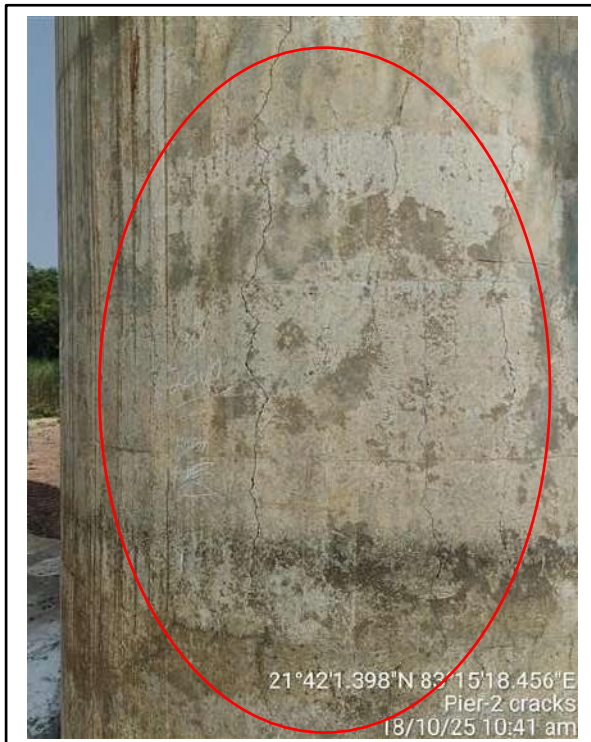
Picture-3 & 4: Cracks on pier surface
