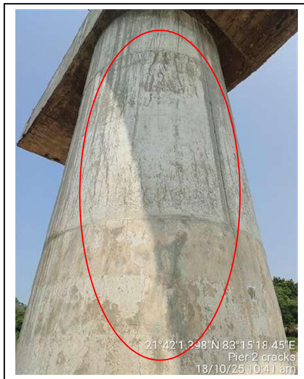
Picture-3 & 4: Cracks on pier surface
