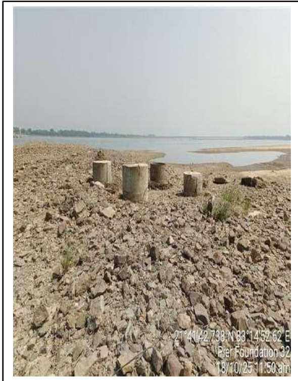
Picture-1: Piles foundation – 32 view
