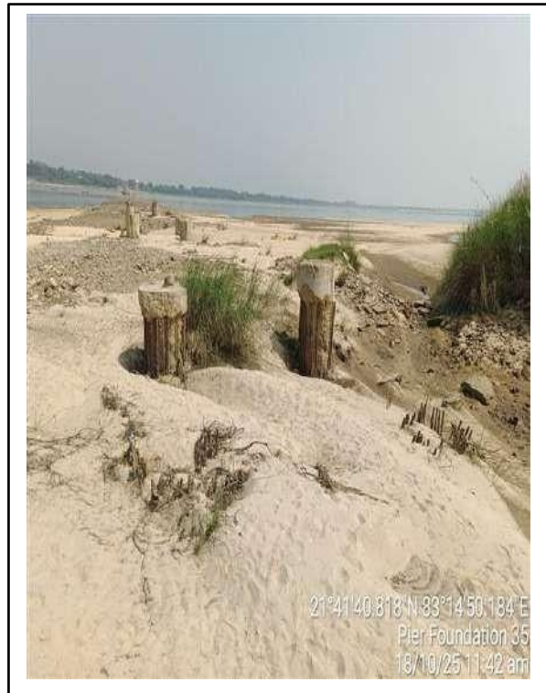
Picture-2: Concrete damage on piles
