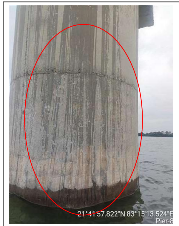
Picture-2: Cracks on pier surface
