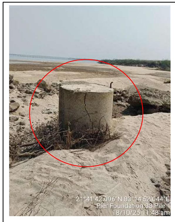
Picture-2: Cracks on pile concrete.
