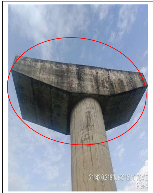
Picture- 5 & 6: Minor cracks & leaching on pier cap.
