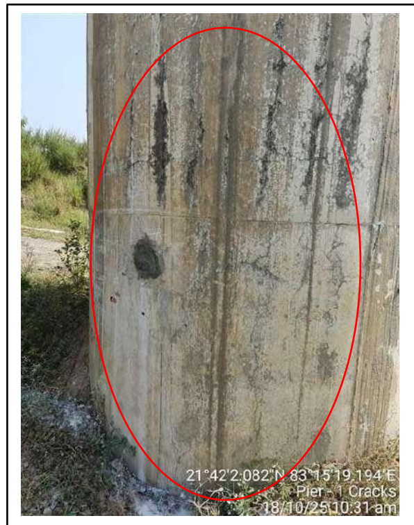
Picture-2: Cracks on pier surface.
