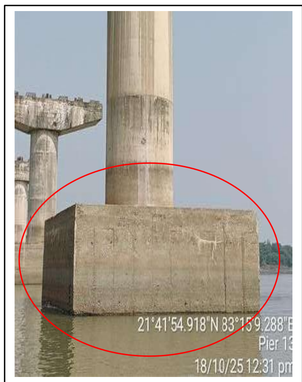
Picture-7 & 8: Cracks on pile cap surface
