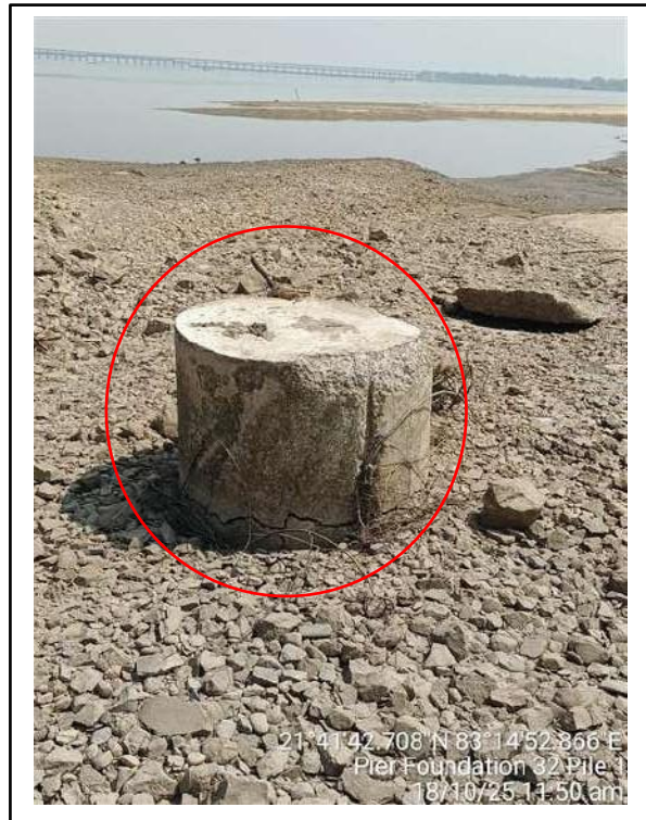
Picture-2: Cracks on pile concrete.
