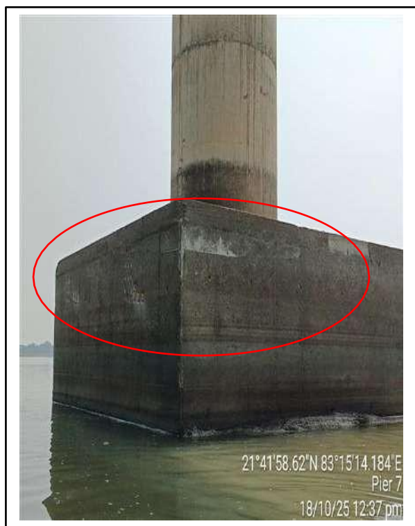
Picture-7 & 8: Cracks on pile cap surface
