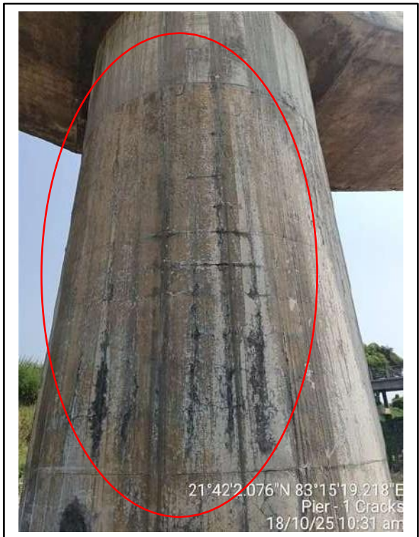
Picture-3: Cracks on pier surface.
