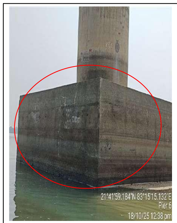
Picture-7 & 8: Cracks on pile cap surface
