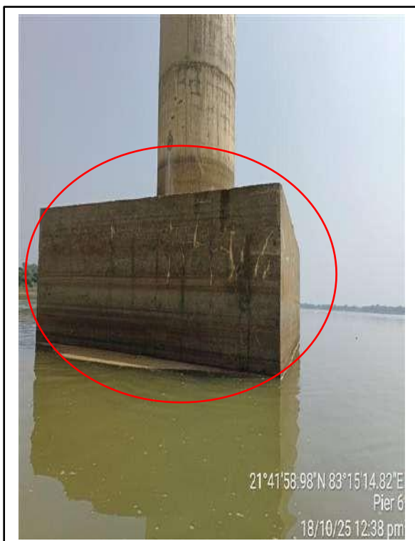
Picture-7 & 8: Cracks on pile cap surface
