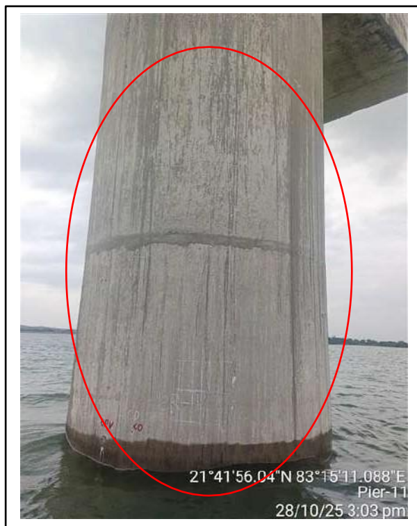
Picture-3 & 4: Cracks on pier surface
