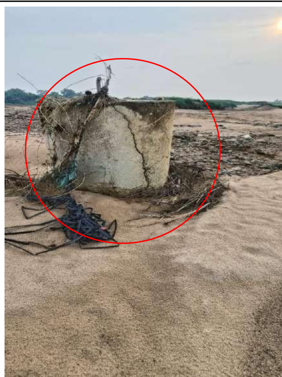
Picture-2: Crack on pile concrete.
