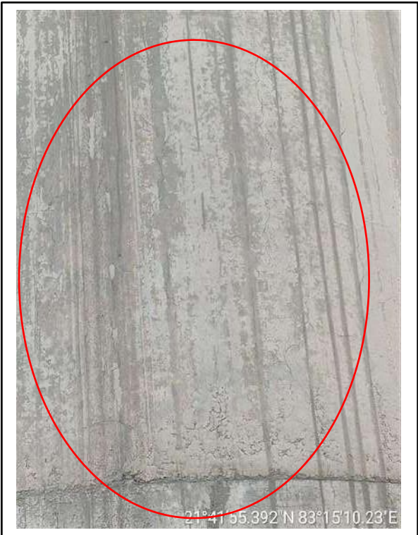
Picture-2: Cracks on pier surface
