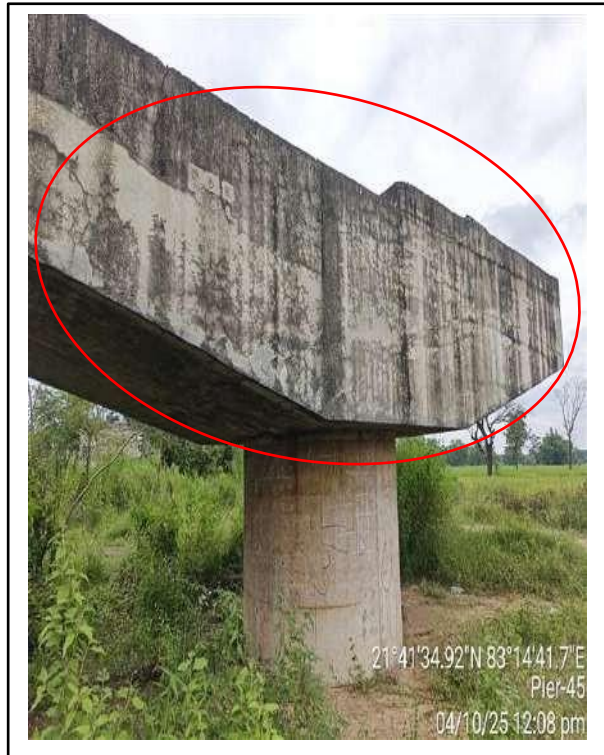
Picture-4: Leaching & minor cracks on cap
