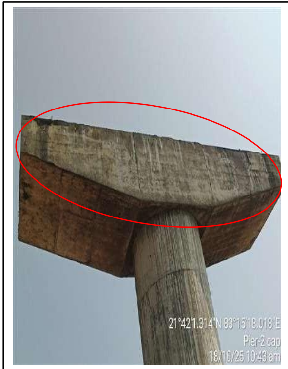
Picture-5 & 6: Surface cracks on pier cap.
