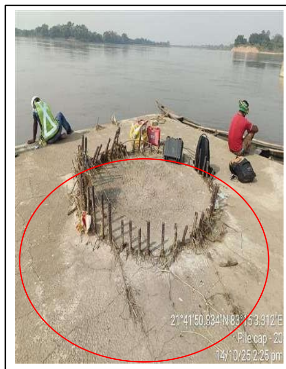
Picture-4: Cracks on pile cap top level.
