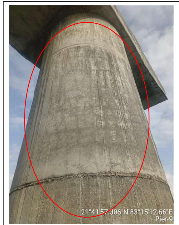
Picture-2: Cracks on pier surface
