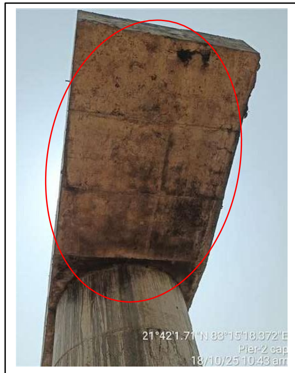
Picture-5 & 6: Surface cracks on pier cap.
