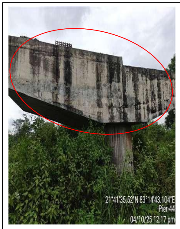
Picture-4: Leaching & minor cracks on cap.
