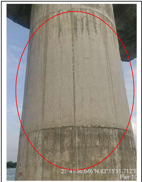
Picture-3 & 4: Cracks on pier surface
