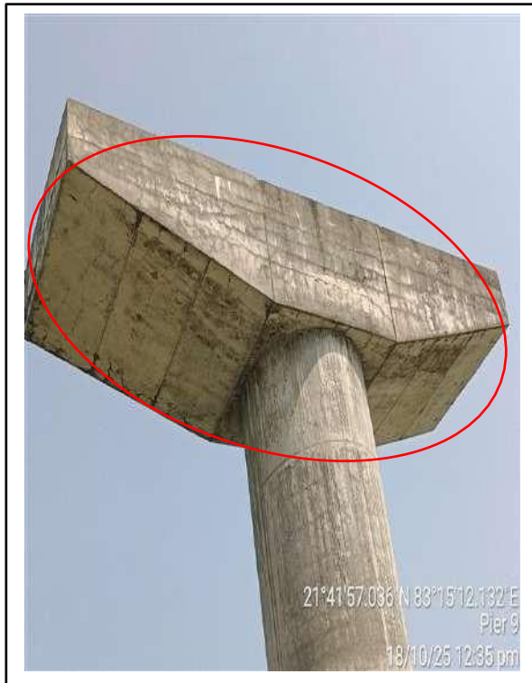
Picture- 5 & 6: Minor cracks, leaching & efflorescence on pier cap.
