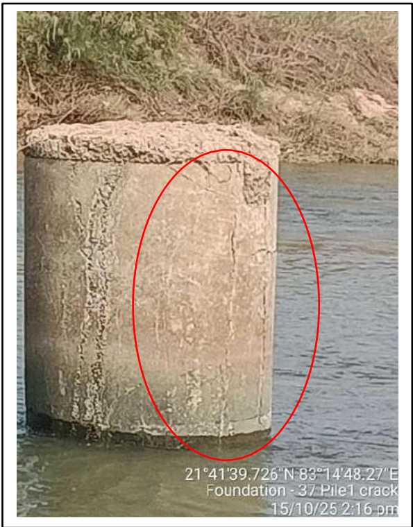
Picture-2: Cracks on pile concrete
