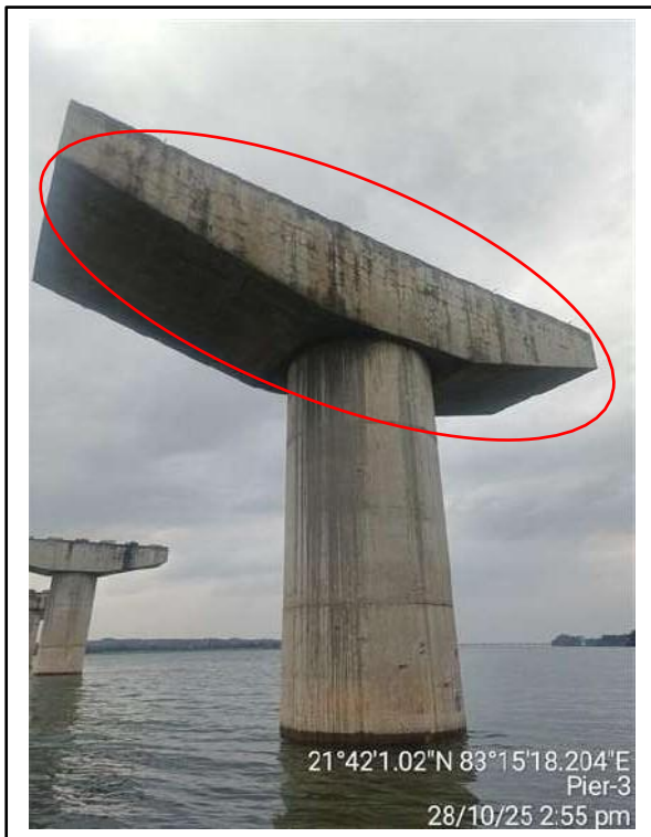
Picture- 5 & 6: Minor cracks & leaching on pier cap.
