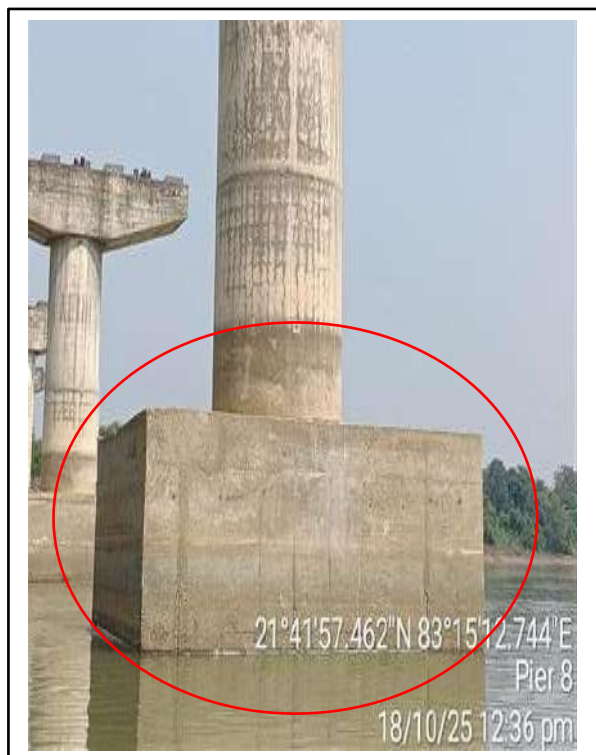
Picture-7 & 8: Cracks on pile cap surface
