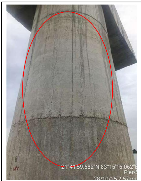
Picture-3 & 4: Cracks on pier surface
