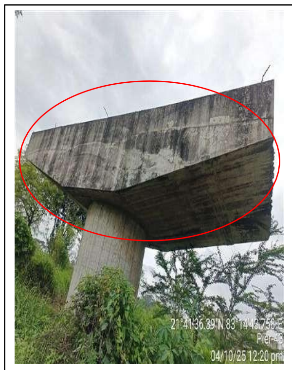
Picture-3: Honeycombs on pier cap bottom face.
