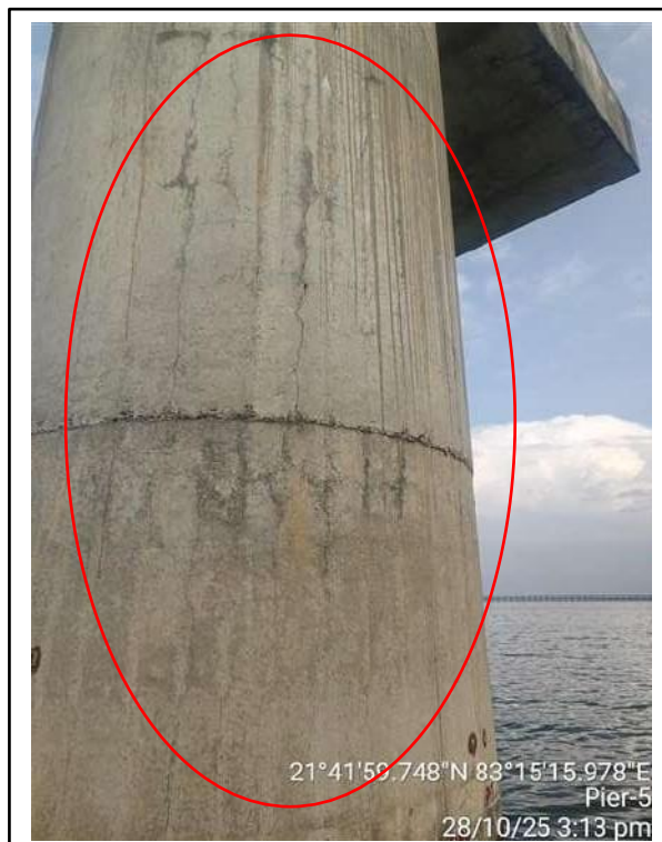
Picture-3 & 4: Cracks on pier surface
