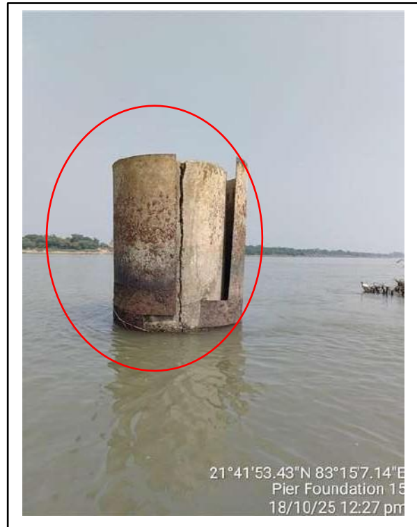
Picture-2: Severe crack on pile concrete
