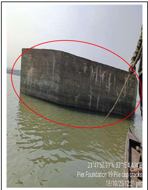
Picture-3: Cracks on pile cap.
