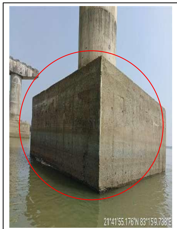
Picture-7 & 8: Cracks on pile cap surface
