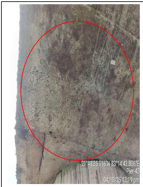
Picture-3: Honeycombs on pier cap bottom face.
