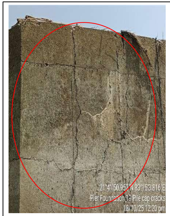
Picture-2: Cracks on pile cap.
