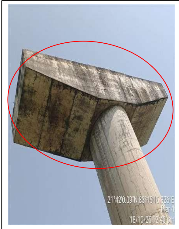
Picture- 5 & 6: Minor cracks & leaching on pier cap.
