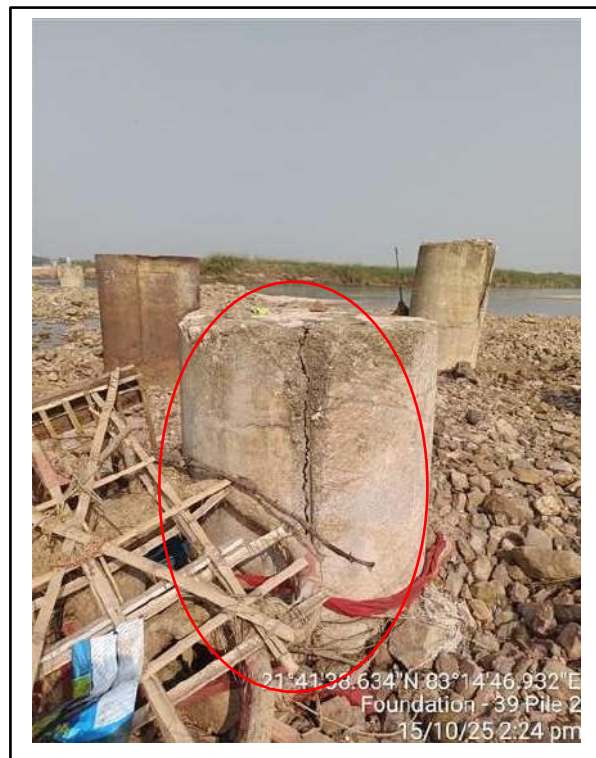
Picture-2: Cracks on pile concrete.
