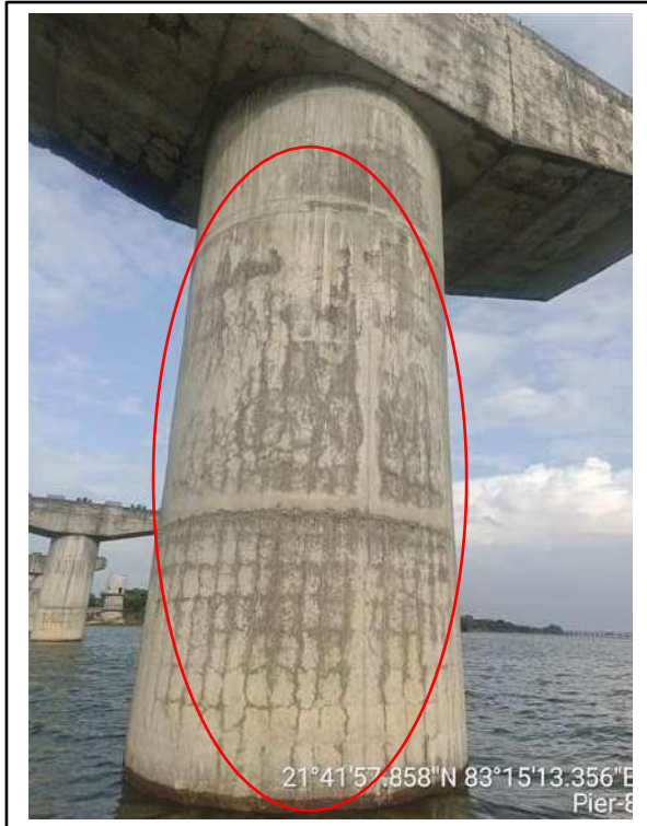
Picture-3 & 4: Cracks on pier surface
