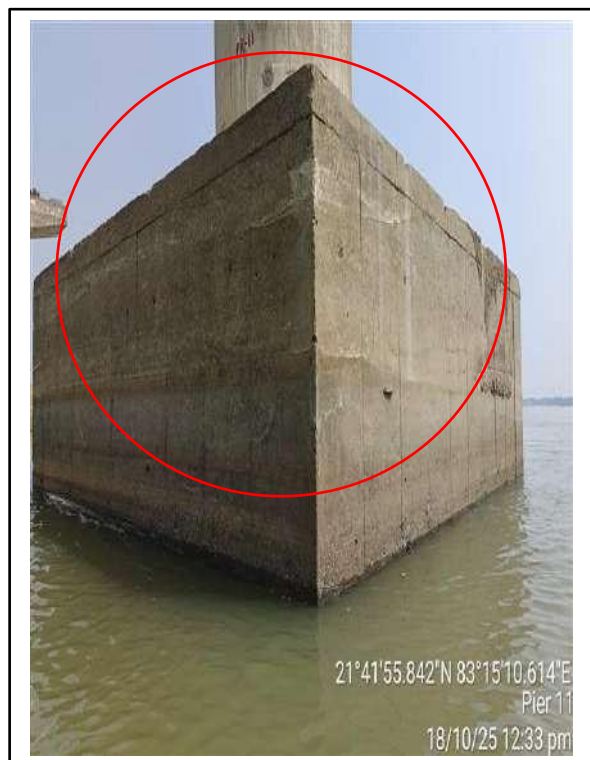
Picture-7 & 8: Cracks on pile cap surface
