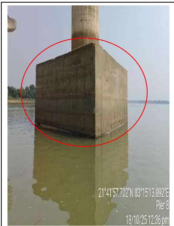
Picture-7 & 8: Cracks on pile cap surface
