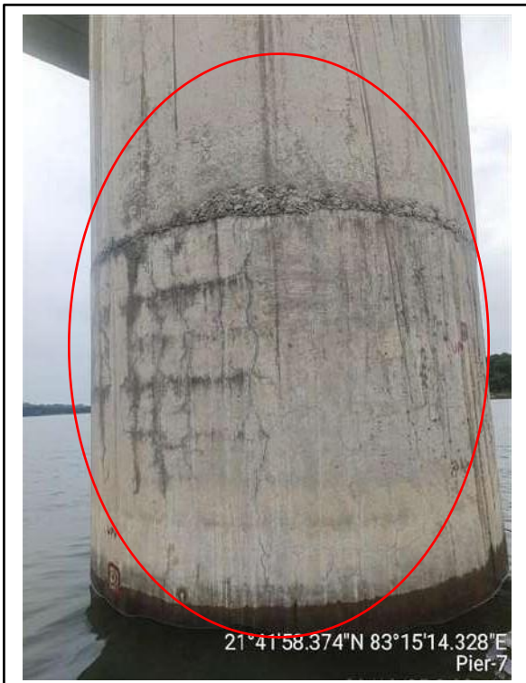
Picture-3 & 4: Cracks on pier surface
