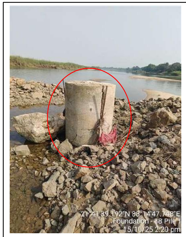
Picture-2: Cracks on pile concrete.
