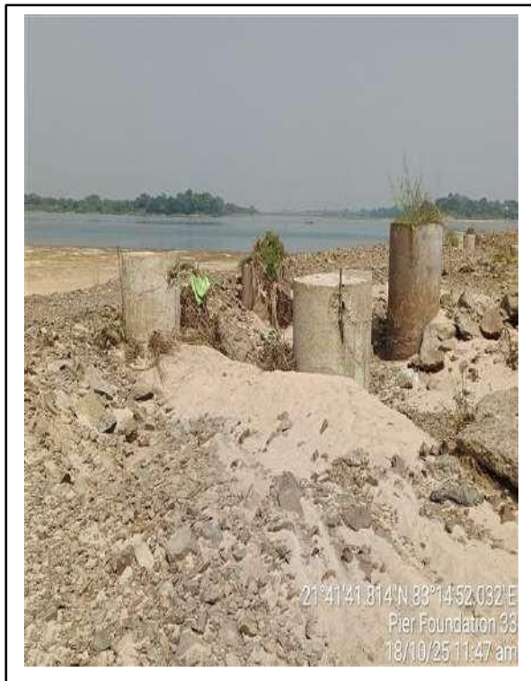
Picture-1: Piles foundation – 33 view
