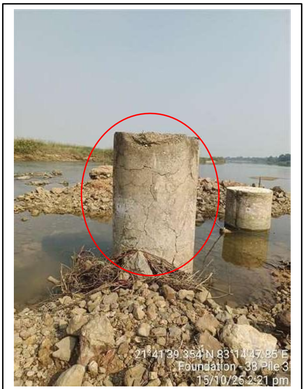
Picture-3 & 4: Cracks on pile concrete.
