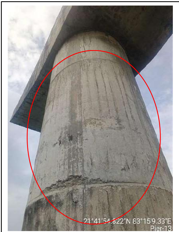
Picture-3 & 4: Minor cracks on pier surface
