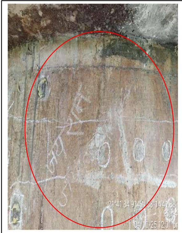
Picture-3: Cracks on pier surface.
