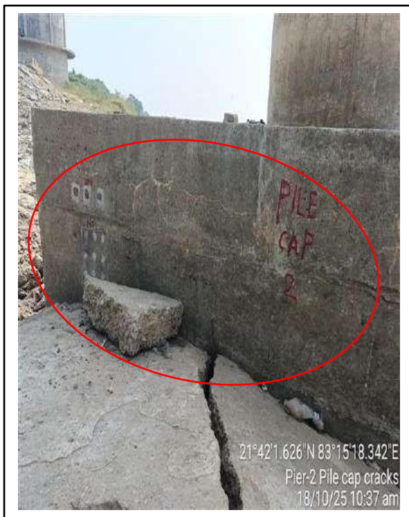
Picture-7 & 8: Cracks on pile cap surface
