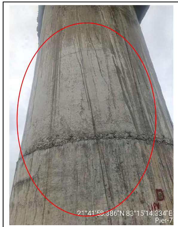
Picture-2: Cracks on pier surface
