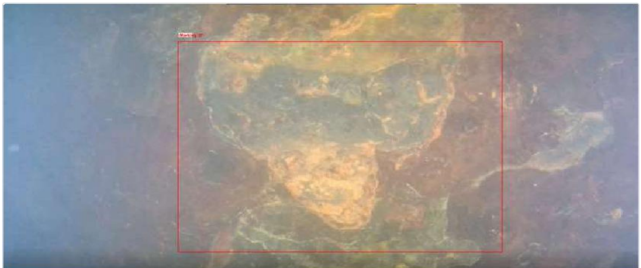
Corrosion and Section loss observed on Piles at various locations.
