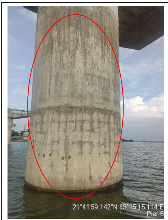
Picture-3 & 4: Cracks on pier surface
