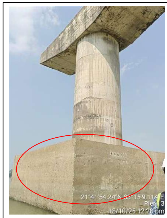
Picture-7 & 8: Cracks on pile cap surface
