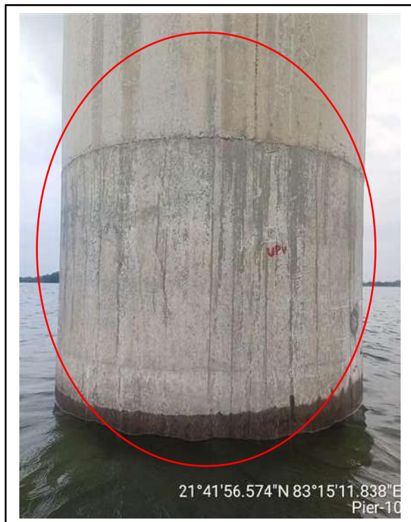
Picture-3 & 4: Cracks on pier surface
