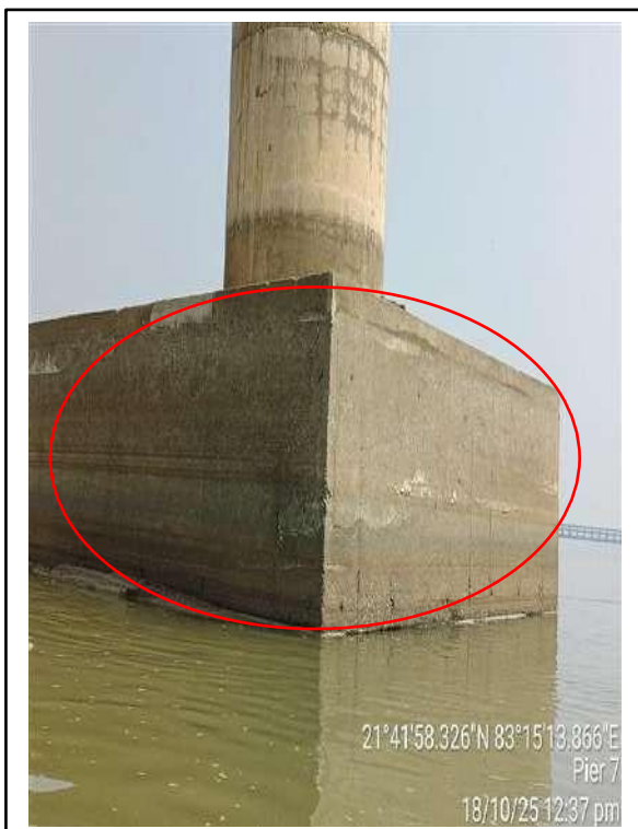
Picture-7 & 8: Cracks on pile cap surface
