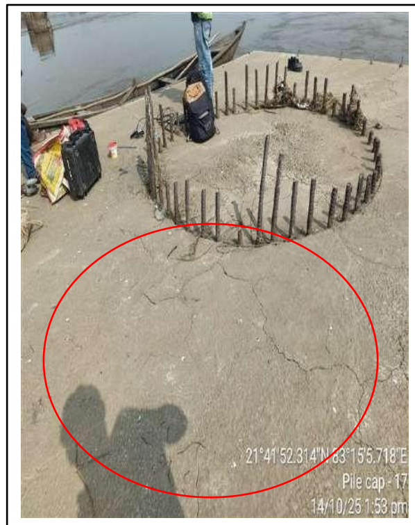
Picture-3 & 4: Cracks on pile cap top face
