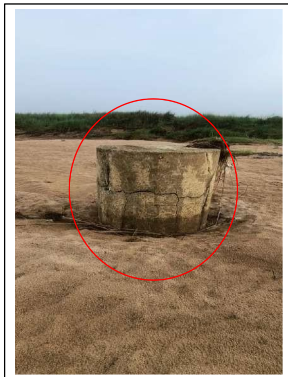
Picture-3: Crack on pile concrete.
