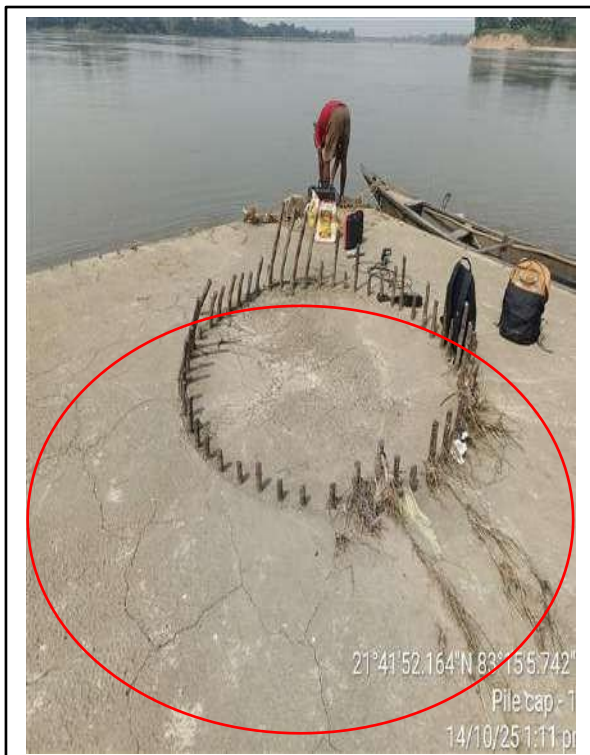
Picture-3 & 4: Cracks on pile cap top face
