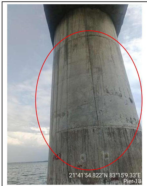
Picture-3 & 4: Minor cracks on pier surface
