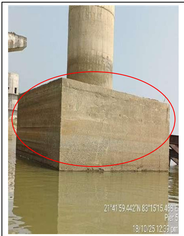
Picture-7 & 8: Cracks on pile cap surface
