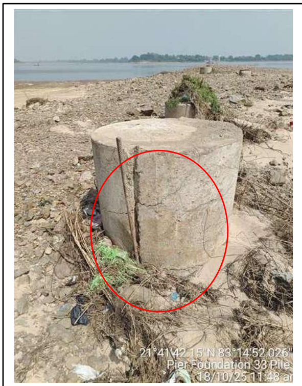
Picture-3 & 4: Cracks and debris on pile concrete
