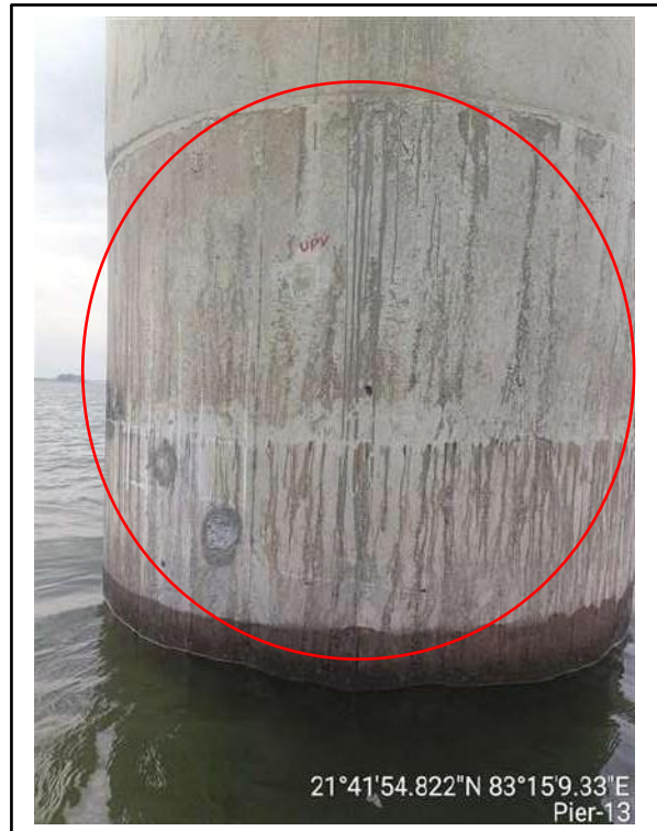
Picture-2: Minor cracks on pier surface
