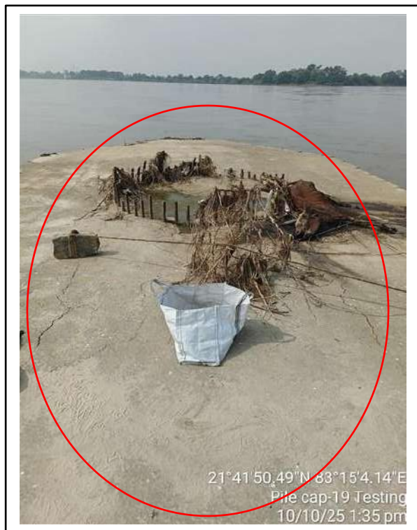
Picture-4: Cracks & Debris on cap.
