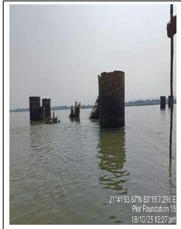
Picture-4: Piles foundation – 15 view
