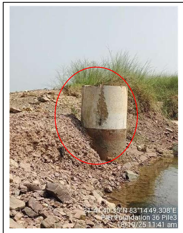
Picture-2: Damage on pile concrete.
