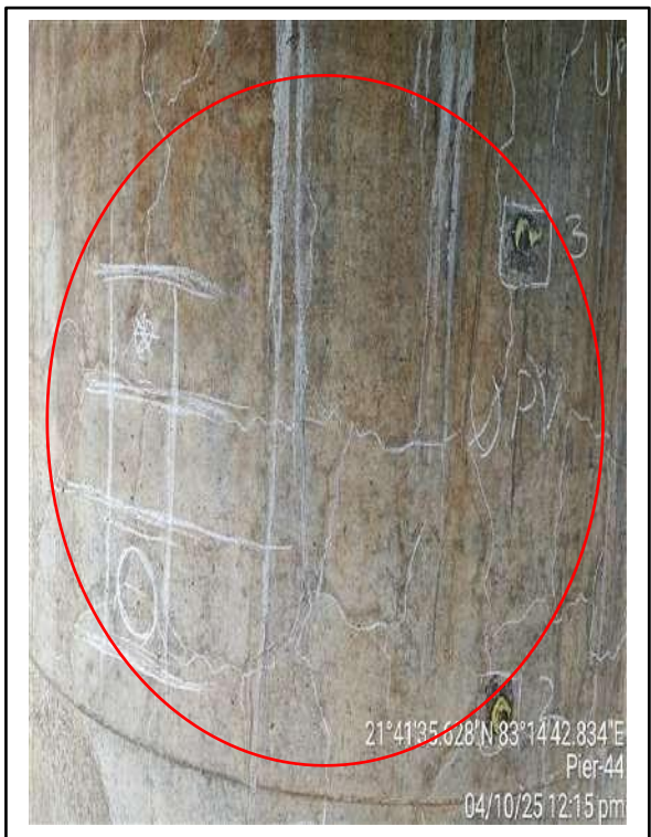
Picture-3: Cracks on pier surface.
