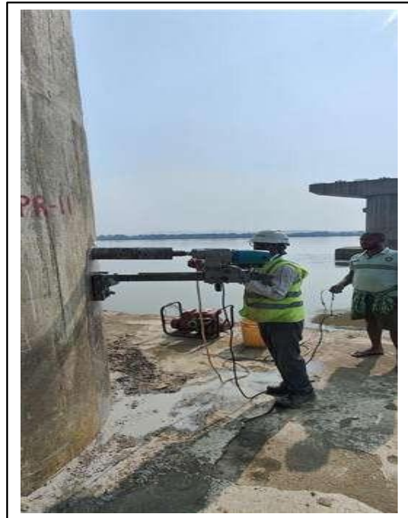
Conducting core cutting test
