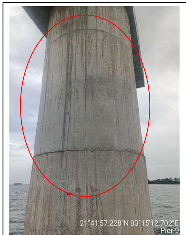
Picture-3 & 4: Cracks on pier surface
