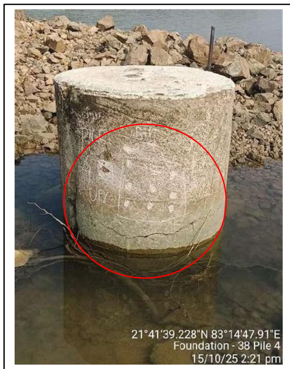
Picture-3 & 4: Cracks on pile concrete.
