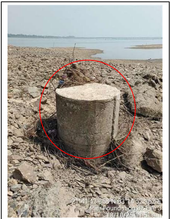
Picture-3: Cracks on pile concrete.
