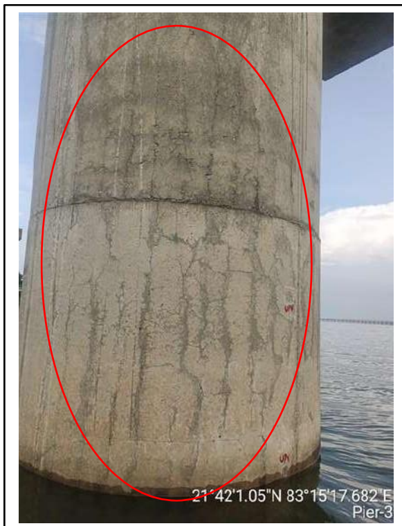
Picture-3 & 4: Cracks on pier surface
