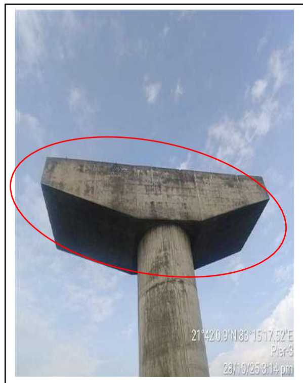
Picture- 5 & 6: Minor cracks & leaching on pier cap.
