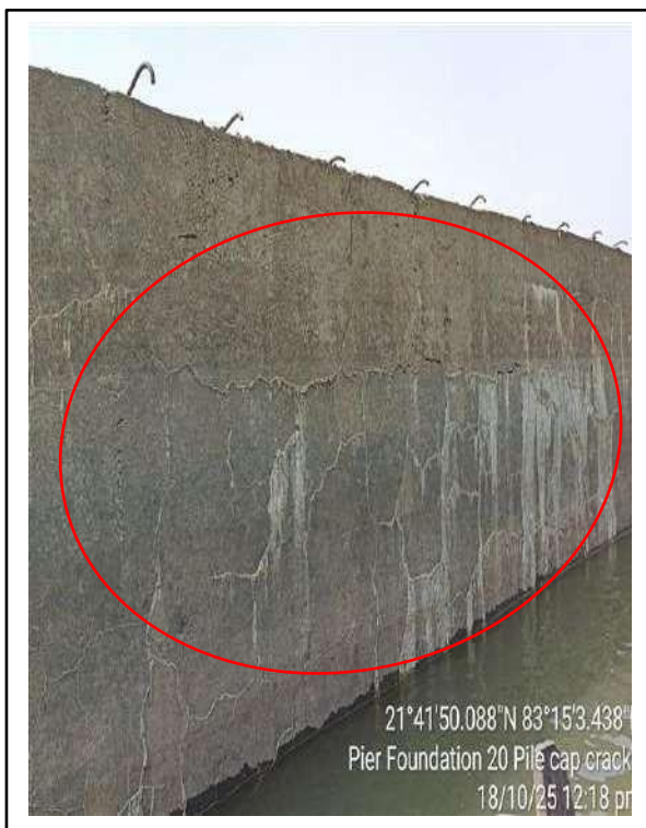
Picture-3: Cracks & Efflorescence on pile side face.
