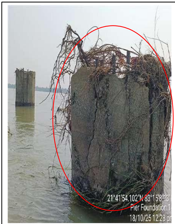
Picture-3: Pile concrete damage.
