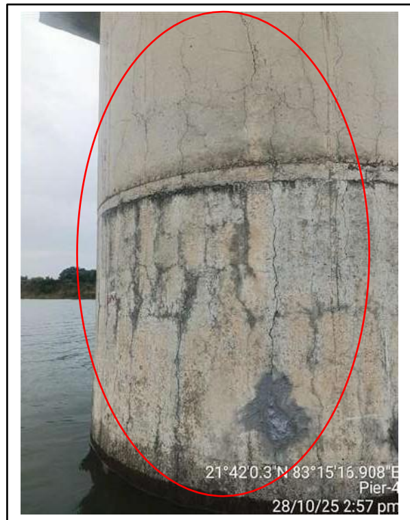
Picture-2: Cracks on pier surface.
