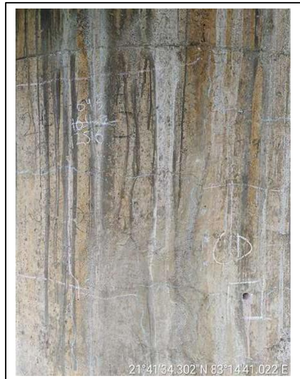
Picture-2: Cracks on pier surface.
