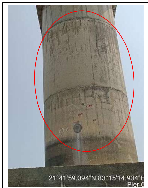
Picture-3 & 4: Cracks on pier surface
