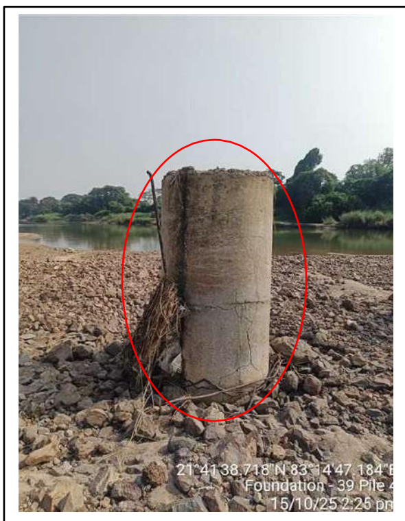
Picture-3: Cracks on pile concrete.
