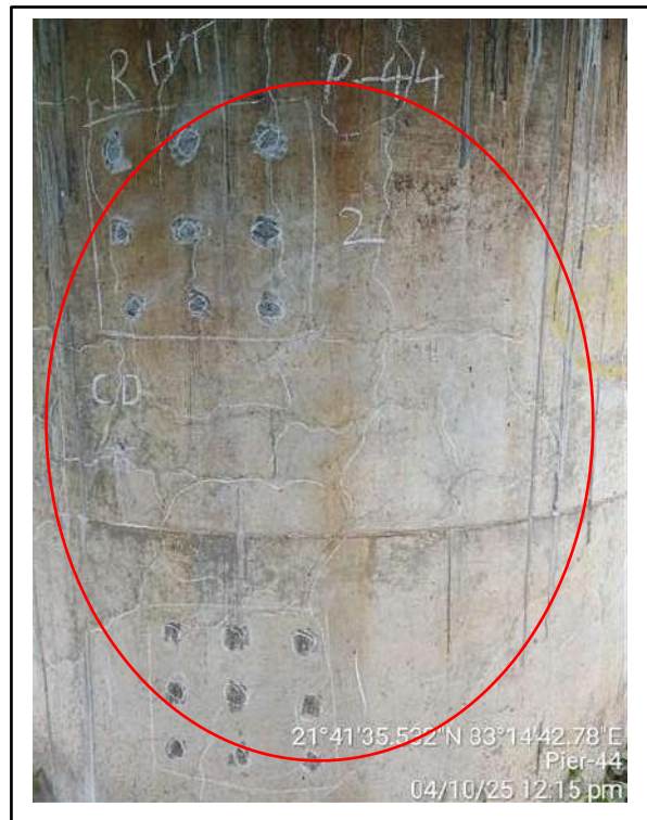
Picture-2: Cracks on pier surface.
