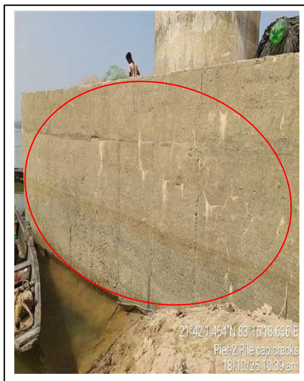
Picture-7 & 8: Cracks on pile cap surface
