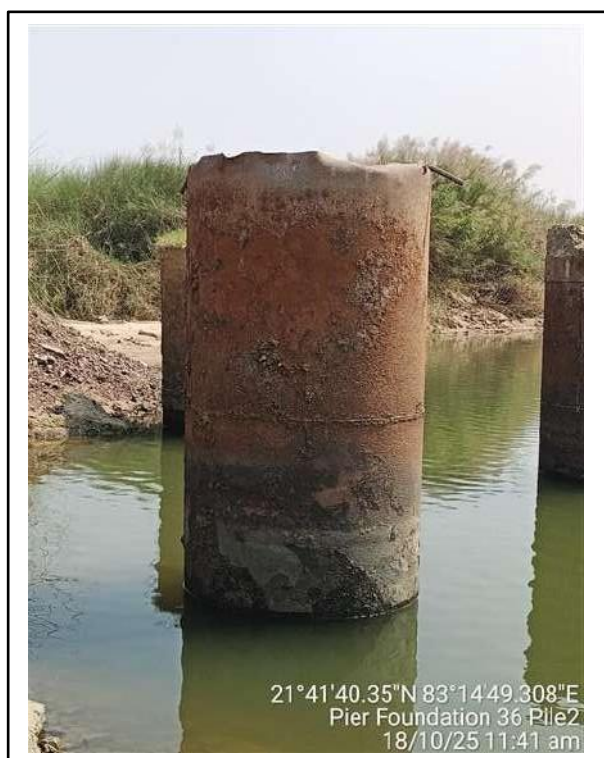
Picture-3: Steel liners for piles above the ground level
