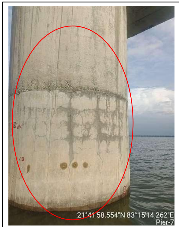
Picture-3 & 4: Cracks on pier surface
