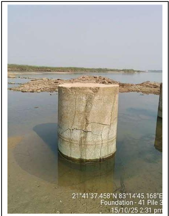
Picture-3 & 4: Cracks on pile concrete.
