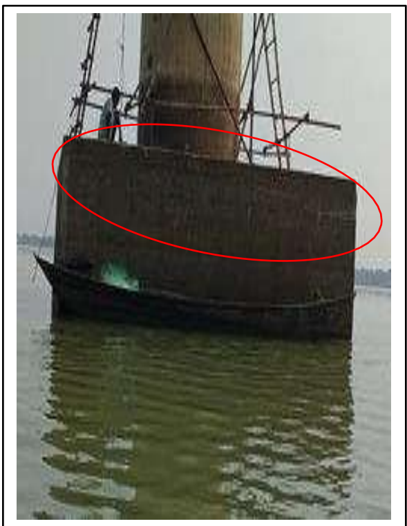
Picture-7 & 8: Cracks on pile cap surface
