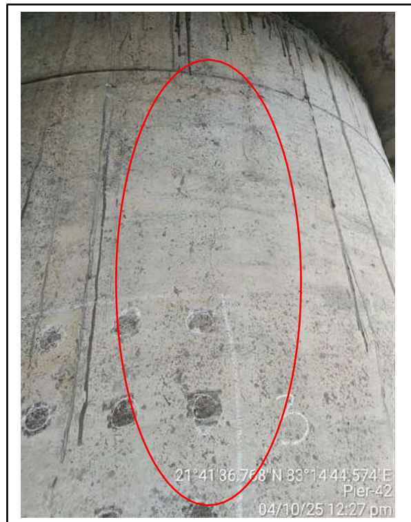
Picture-2: Cracks on pier surface.
