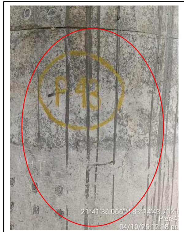
Picture-2: Cracks on pier surface.
