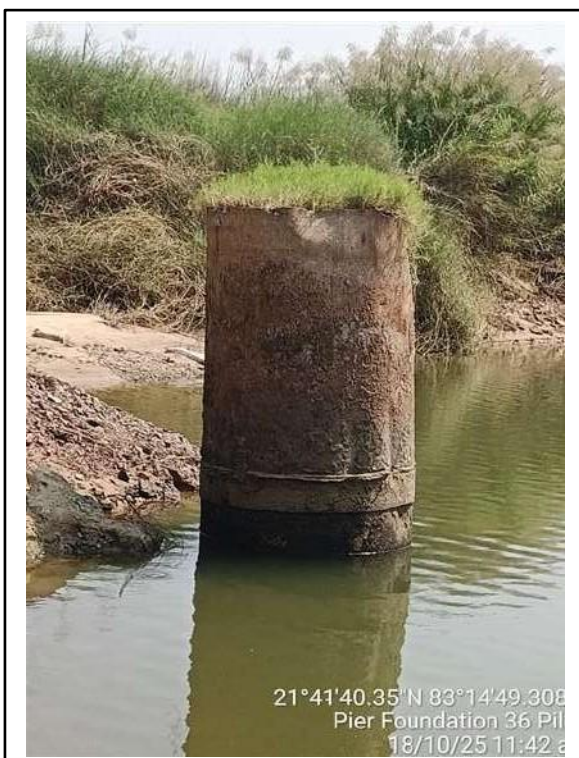
Picture-3: Steel liners for piles above the ground level
