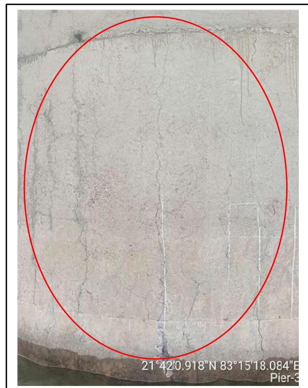
Picture-2: Cracks on pier surface.
