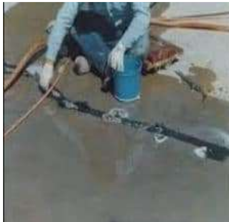
Fig. 2: Sealing Cracks between Ports
