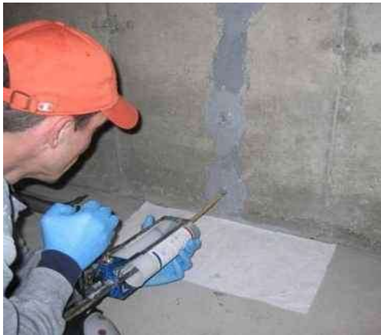
Fig. 5: Pressure Injection Grouting
