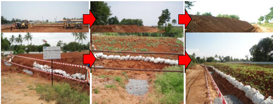
Figure 2: Process of Top Soil Preservation
